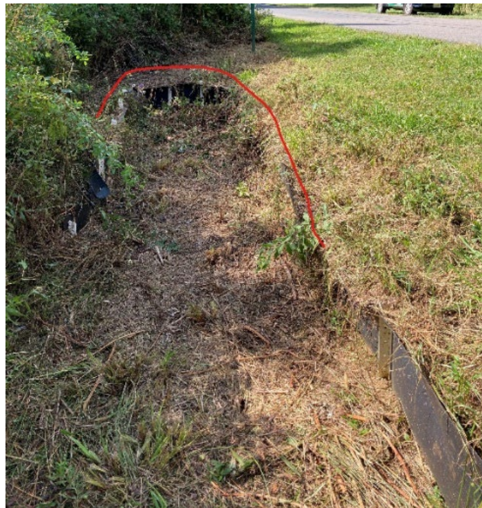
Figure 11. Curved turtle fence end to deter turtle from going around the fence. This barrier is built into the slope so it is at grade on the roadside so that an animal that is on the road is not trapped and may drop over the lip to the wetland but not move from wetland to the road.
