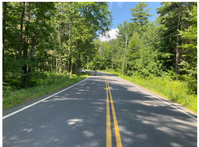
VIEW OF ROAD
