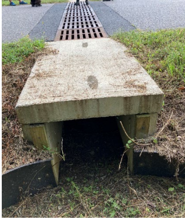
Figure 14. A dry culvert with a grated cover.
