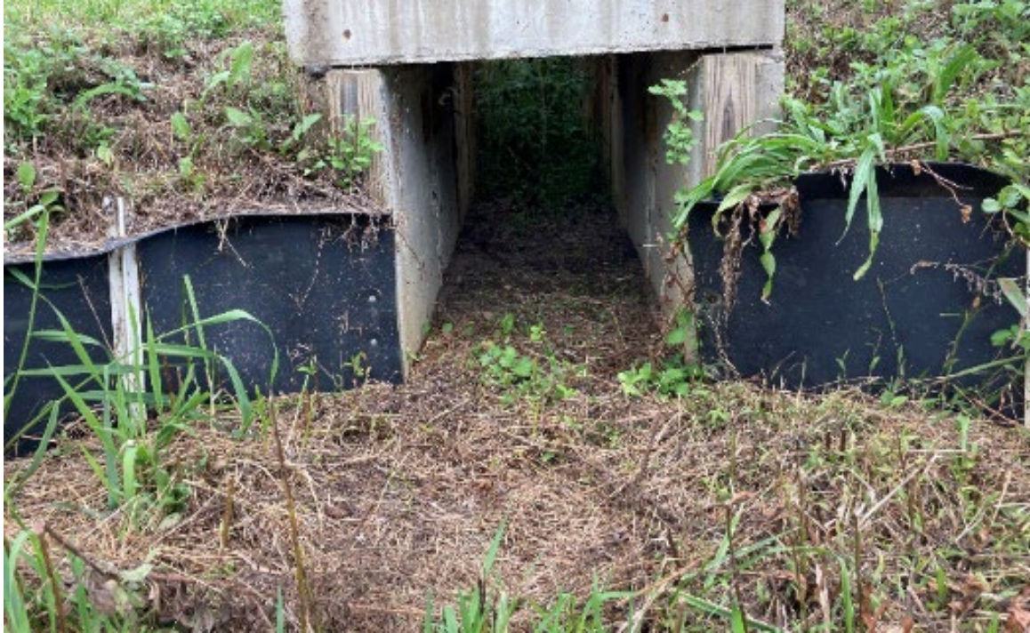
Figure 17. Example of a dry passage culvert.
