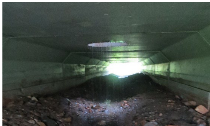
Figure 13. A grate in the shoulder of a roadway provides light to a culvert; installing the grate in the shoulder of the road allows it to be below road grade improving snowplow safety.
