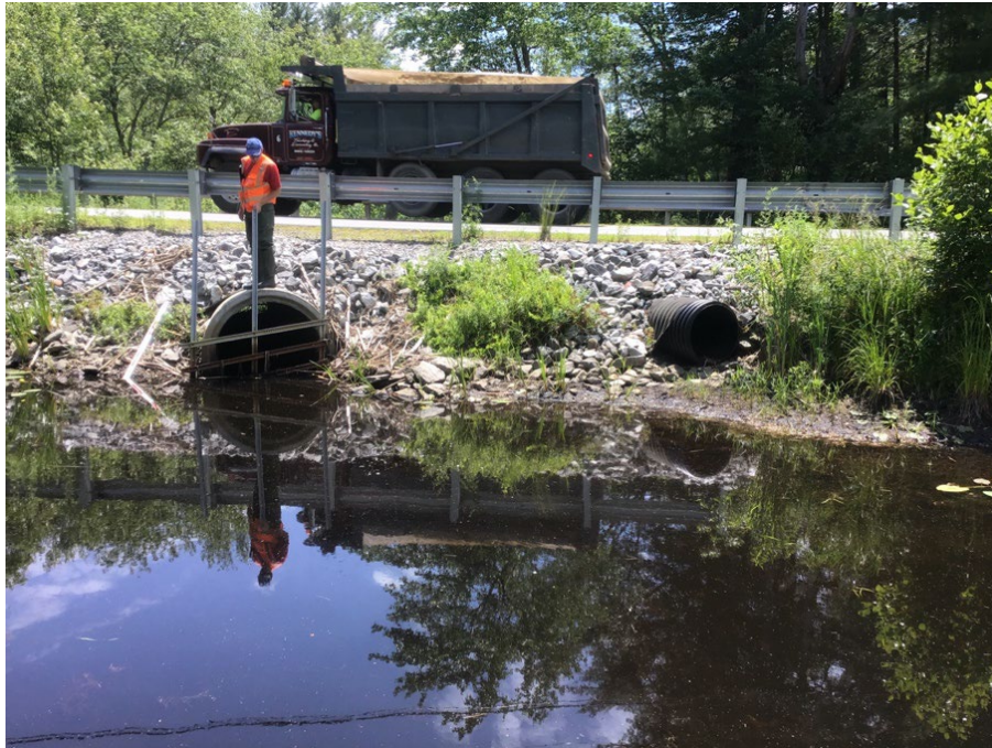
Figure 5. Relatively steep embankment slope by the culvert inlets with rip rap on the embankment, reducing riparian continuity. In this instance, passage from the water to the road is relatively difficult compared to Figure 6 and would likely take more energy, or potentially be a barrier.
