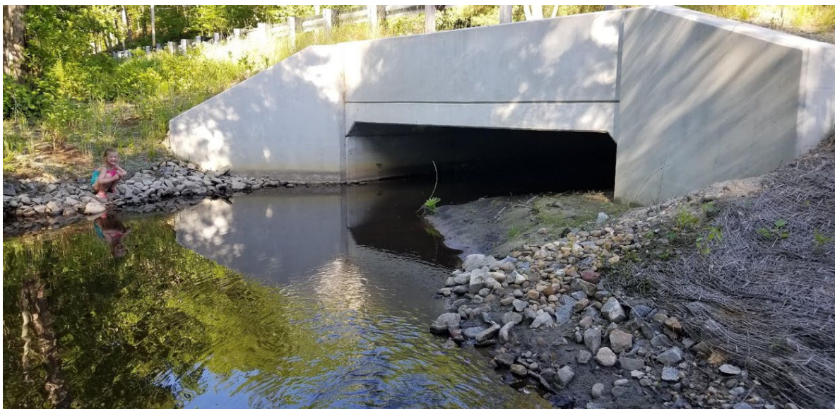
Figure 7. Lack of riparian continuity leading into and through a structure due to cobble and rip rap placed on banks.
