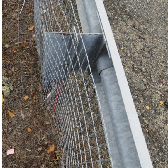
Figure 12. Turtle fence installed behind an existing guardrail.
