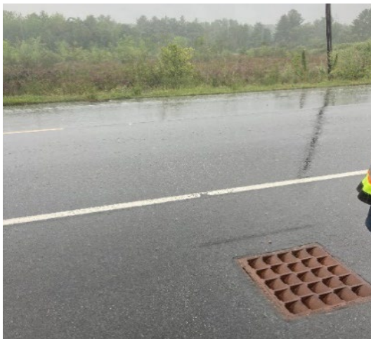
Figure 13. A grate in the shoulder of a roadway provides light to a culvert; installing the grate in the shoulder of the road allows it to be below road grade improving snowplow safety.
